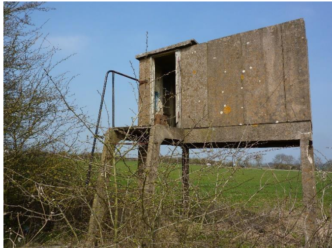
FIGURE 9 AN ORLIT 'B' ROYAL OBSERVER CORPS POST, AN AIRCRAFT REPORTING POST, IS LOCATED IN BUCKDEN
